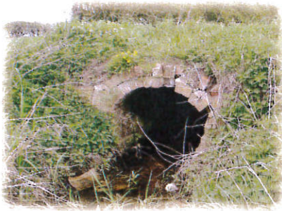
Drainage Culvert on Prestwick Carr
