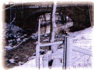
Looking back at Dissington Bridge
