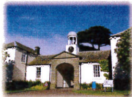
Arch into courtyard at Kirkley Hall
